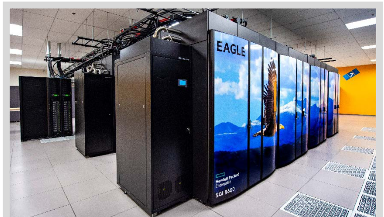
NREL researchers used the Eagle supercomputer to visualize flow fields for the IEA Wind Task 29 validation campaign, which will enable new designs to help reduce the levelized cost of wind energy. Photo by Dennis Schroeder
