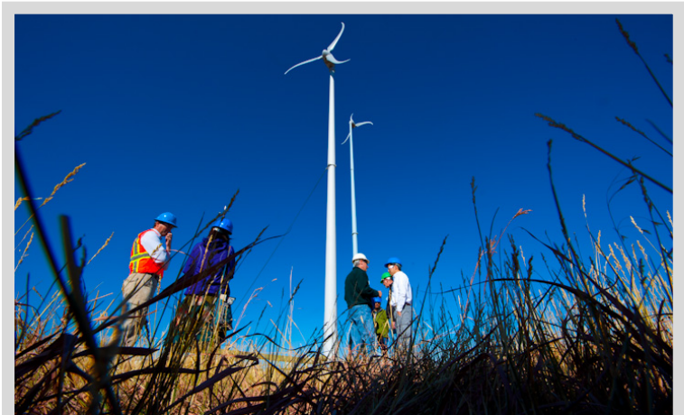
Minimizing material use and manufacturing cost while increasing annual energy production is important for the continued adoption of small wind turbines like these Southwest WindPower Skystream turbines shown here on NREL's Flatirons Campus. NREL researchers used the FAST aeroelastic model of a 2.6-kW turbine in the foreground as one turbine design option in their research published in Wind Energy . Photo by Dennis Schroeder, NREL
