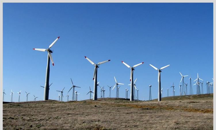
Many wind turbines installed decades ago are reaching the end of their lifetimes, which has prompted NREL researchers to understand what can be done with old turbine parts. NREL photo
