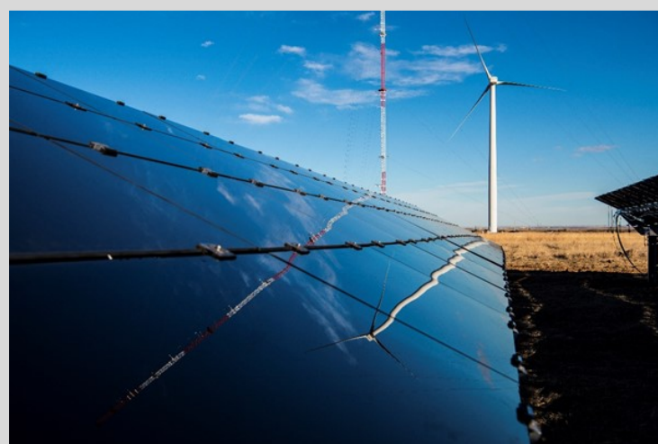
Among other findings, NARIS describes how an integrated grid can be reliable, economically efficient, and enable high contributions of renewable resources throughout the continent. Photo by Dennis Schroeder, NREL
