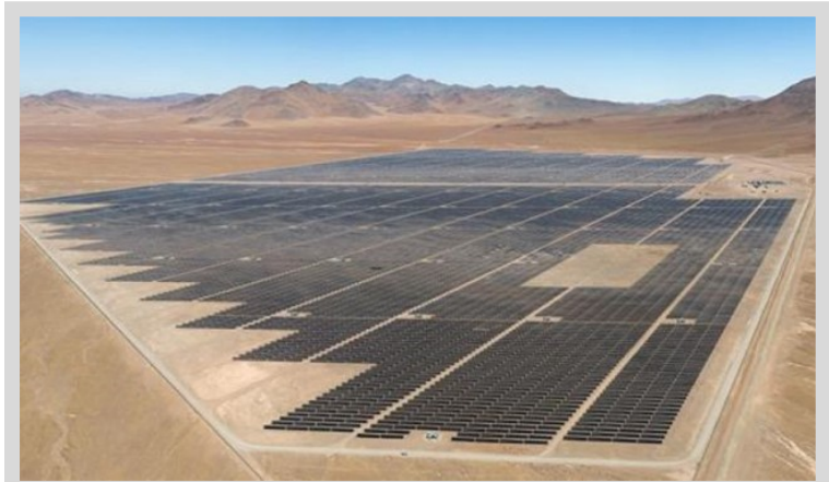
Grid-scale utility assets and numerous renewable energy and storage technologies could work together to provide stability to the power grid. Photo courtesy of First Solar
