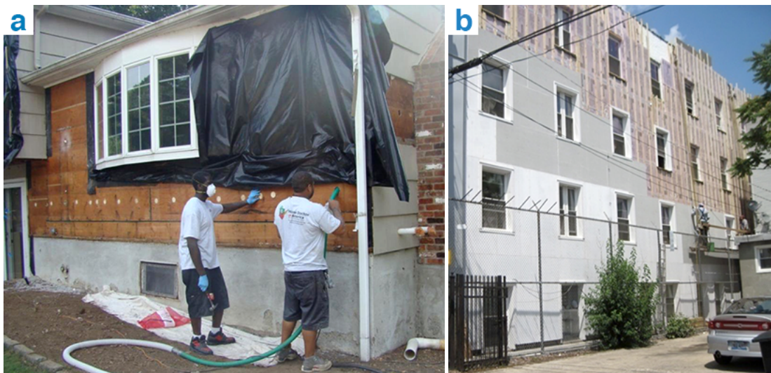
Figure 7. Drill-and-fill insulation (a) reduces heat transfer through walls by adding insulation to cavities between studs through small filling holes in each stud bay; overclad insulation retrofits (b) add one or more layers of insulation (typically rigid foam insulation) on top of the existing exterior facade; the insulation is covered by new exterior finishing layers.
