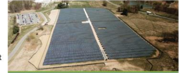
A nearly 15,000-panel solar PV array was installed under an ESPC ESA at the U.S. Department of Commerce's National Institute of Standards and Technology (NIST) in Gaithersburg, Maryland. The installation will be privately owned for the 20-year ESPC ESA term for tax incentive purposes and NIST will purchase the electricity produced. The array is predicted to save NIST a minimum of $3.5 million in its first 20 years of operation. Photo courtesy of NIST.
