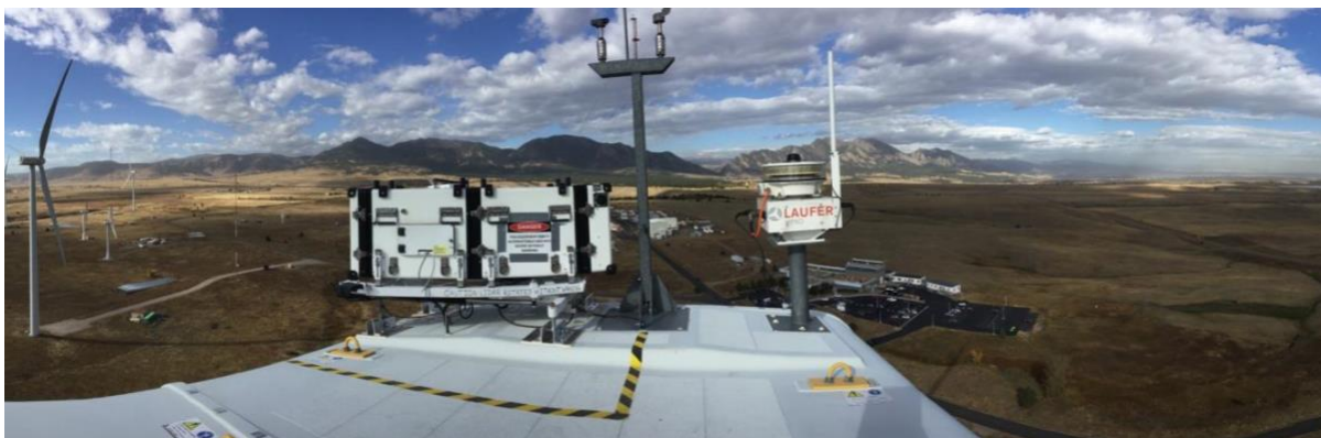
Figure 4: Photo showing the lidar, wind vane, and cup anemometers mounted to the back of the wind turbine nacelle.
