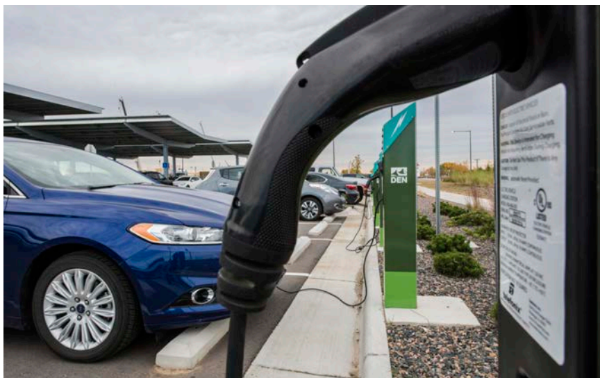
Public charging stations typically include one or more “Level 2” units and may include “DC Fast Charge” units as well. Photo by Dennis Schroeder, NREL 48757.
