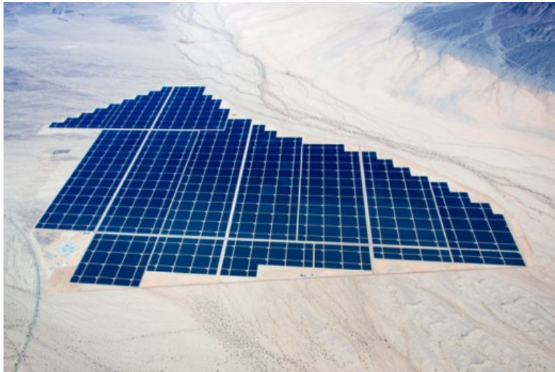
550 MW CdTe solar farm in the Mojave desert Photo: First Solar
