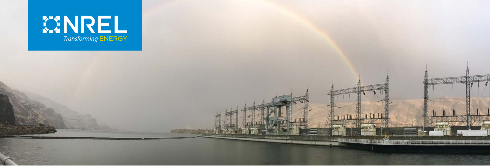
Rainbow over the Rocky Reach Dam in Washington State. Photo from Katelynn English, U.S. Department of Energy
