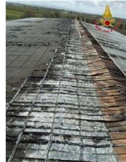
Example of PV fires in Italy. Fiorentini et. al., PVRW 2020.
