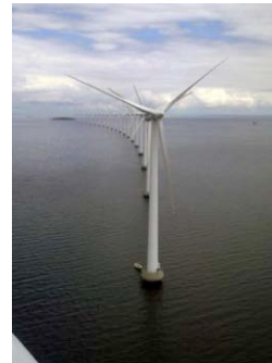
Photo from HC Sorensen, NREL 17855
