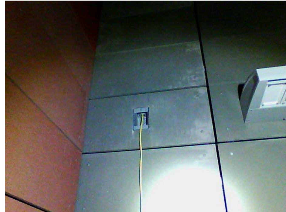
Poor conduit seal at J-box installation
