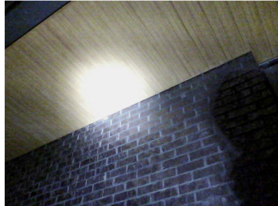
Poor seal or thermal break at exterior roof line
