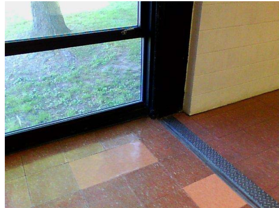
Leakage through a window (this is typical)
