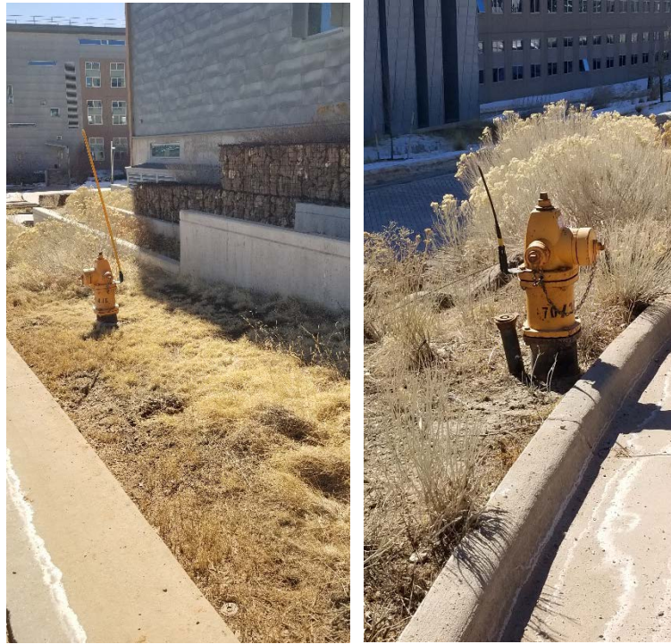
Figure C-7. Hydrants were generally kept clear of vegetation that would prevent their use in a wildfire; however, shrubs should be trimmed on right
