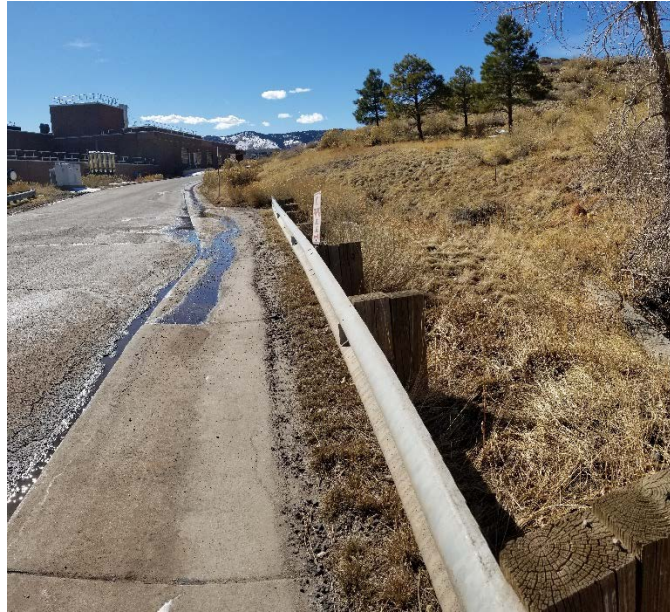
Figure C-5. Roadsides should be mowed for a width of 10 feet from road edge
