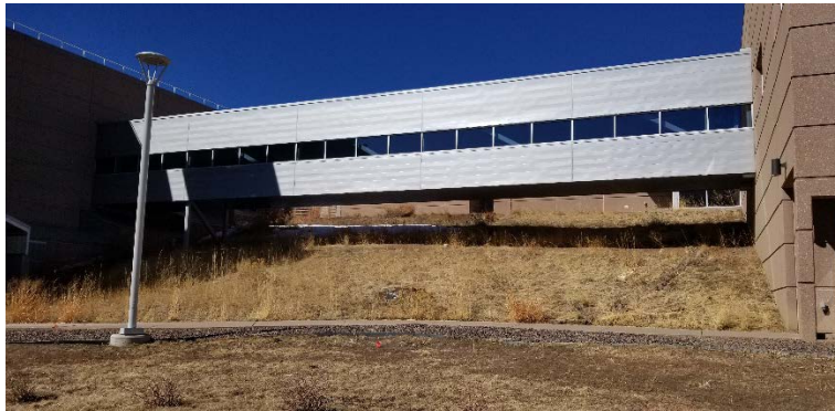
Figure C-9. Not all structures currently have grass mowed within 30 feet of the building edge
