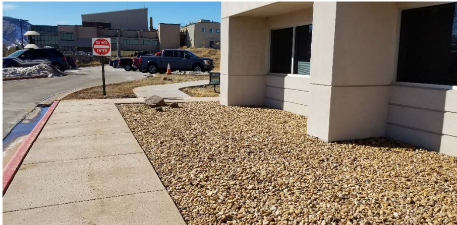
Figure C-1. Excellent example of a noncombustible zone
