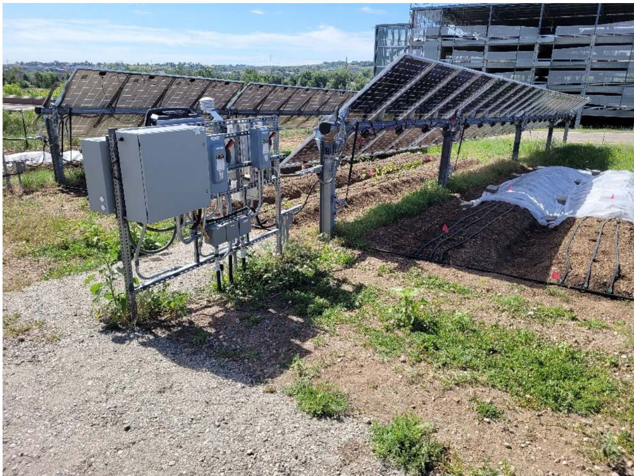
Figure 19. Placement of solar technology equipment on an agrivoltaic site.
