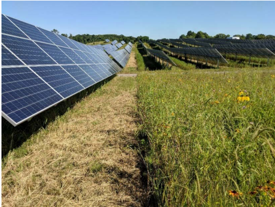
Figure 18. Different types of vegetation under the array vs. outside of the array (top) as well as targeted mowing strips adjacent to panels to avoid panel shading (bottom) from InSPIRE research sites in Minnesota.
