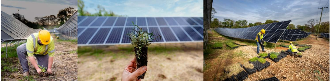
Figure 26. Planting plugs for ecosystem services and beneficial habitat could accelerate vegetation establishment, albeit at a higher cost.
