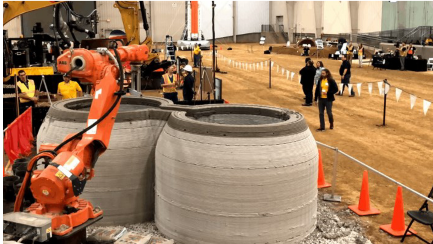
ACTUAL CONSTRUCTION AT FINALS IN PEORIA, ILLINOIS
