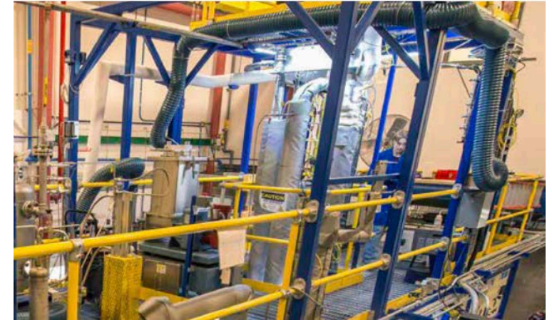
Davison Circulating Riser* at NREL
