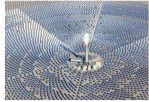
The heliostats considered for this investigation consist of a grid of mirror facet panels mounted on a motorized system
