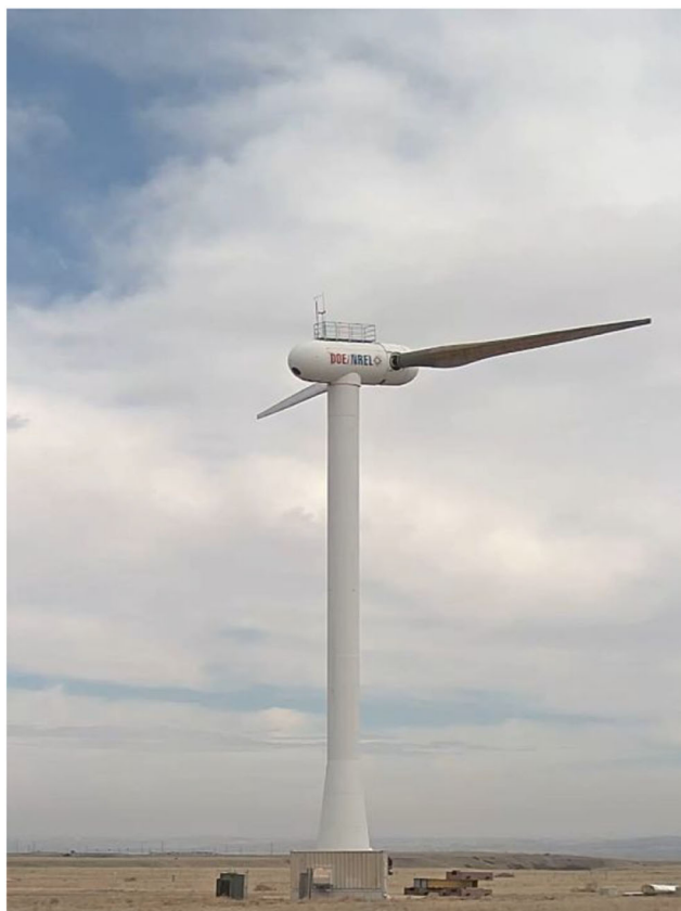
FIGURE 1 The SUMR-D blades mounted on the two-bladed CART-2 at the NREL FC and placed in parked conditions
