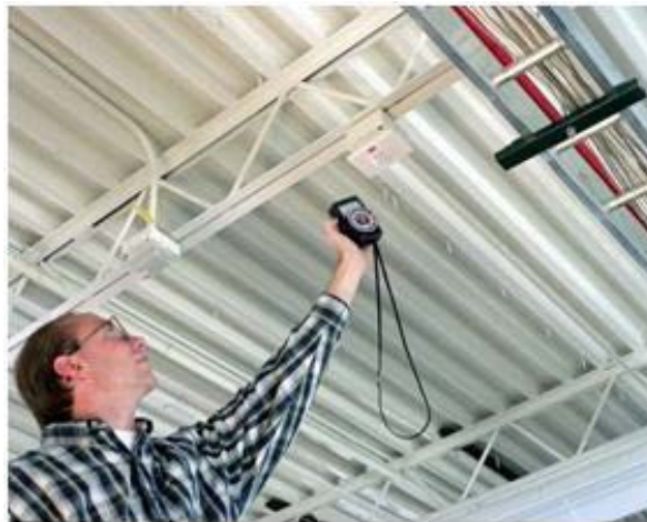
Figure 35. A researcher checks the quantity of daylight and the accuracy of the lighting sensors Photo by NREL/PIX 05171
