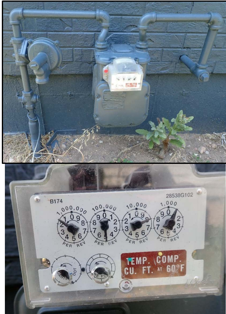
Figure 62. Example of a utility gas meter. In this case, the lower left dial measures \frac{1}{4} cubic foot of gas per revolution. Note that the meter has temperature compensation and measures cubic feet of gas at 60°F
