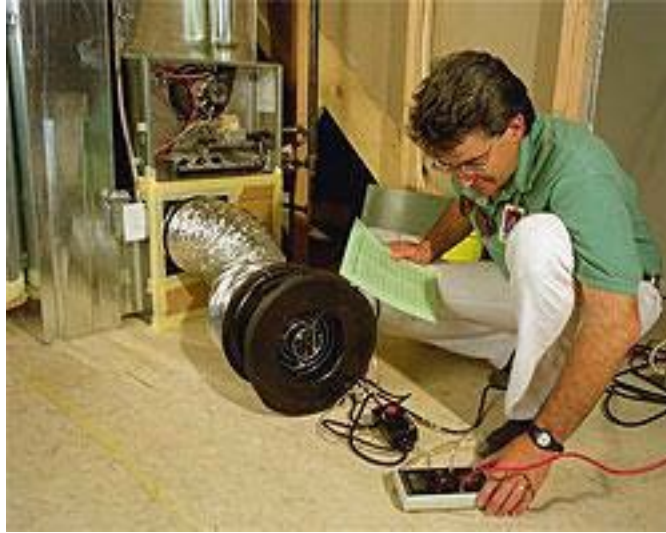
Figure 7. A duct pressurization test in process
