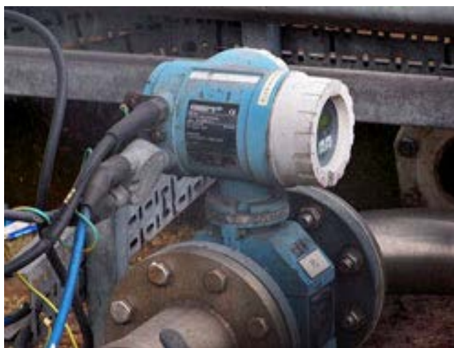
Figure 49. A magnetic flow meter in use at a brewery
