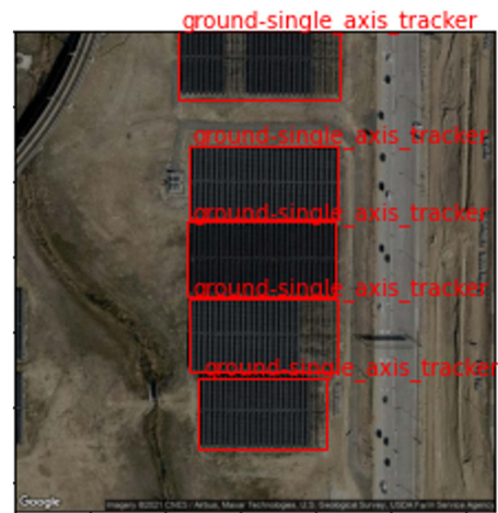
Fig. 1. Labeled satellite image, showing single axis tracker installations.
