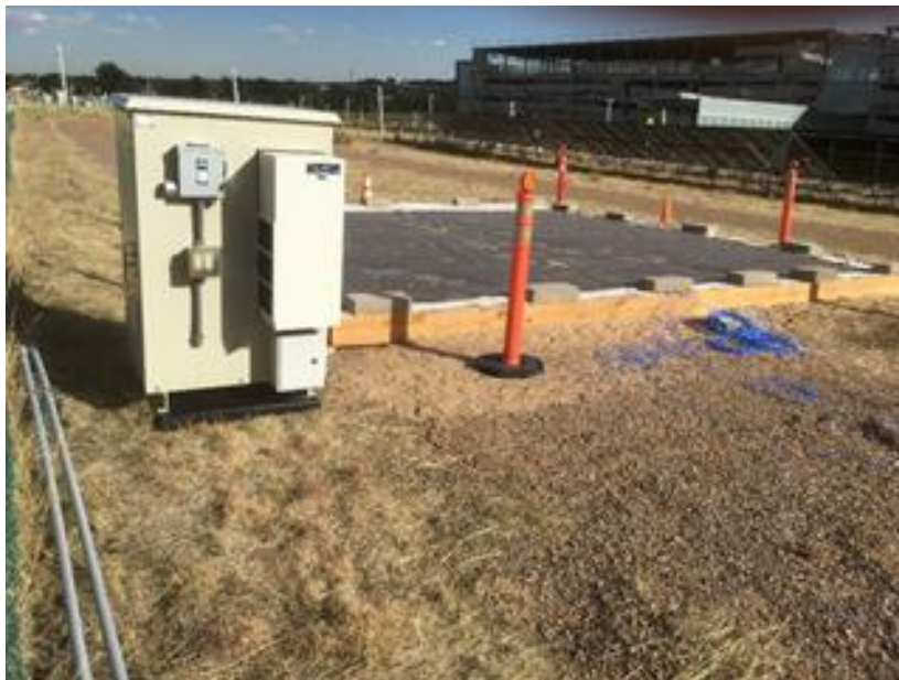
Figure 1. 32 PV Modules installed at NREL's Outdoor Test Field
