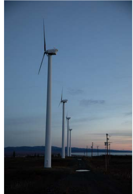
Photo by Werner Slocum, NREL
