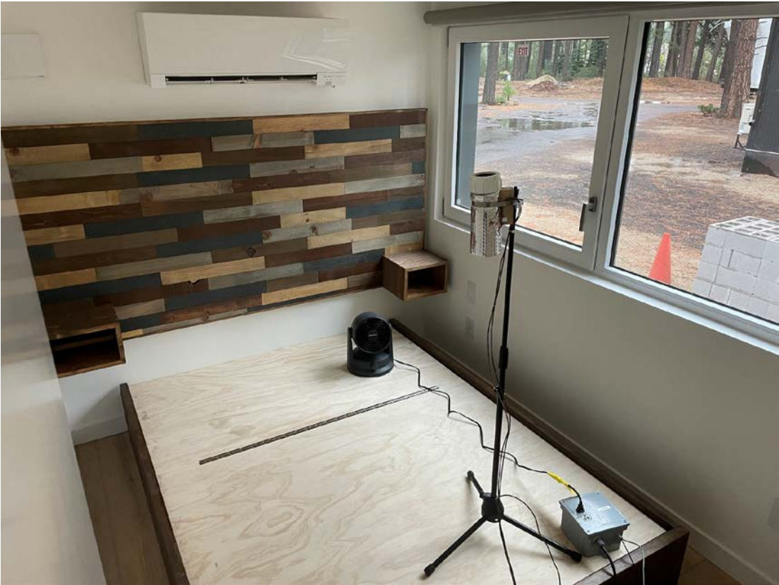
Figure 12. Space heater, controller/watt node, and aspirated thermocouple in the downstairs bedroom
