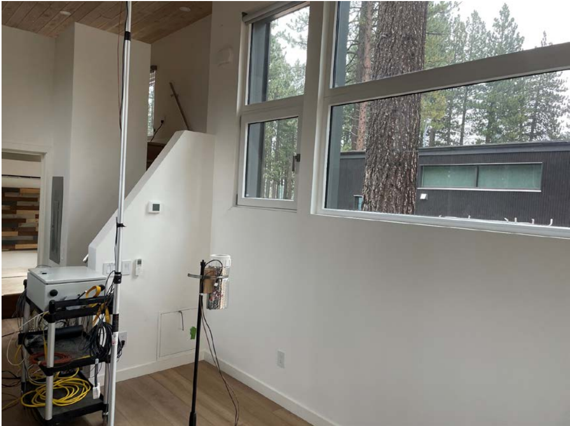
Figure 14. Thermocouple array for measuring thermal stratification (left) and aspirated thermocouple (center) in the main living area
