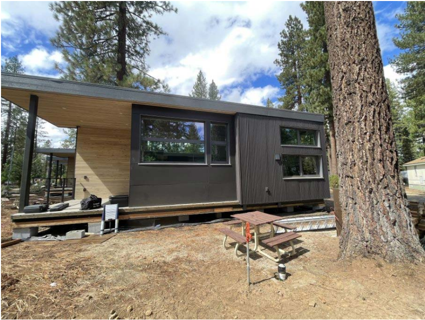
Figure 3. East side view of the test house
