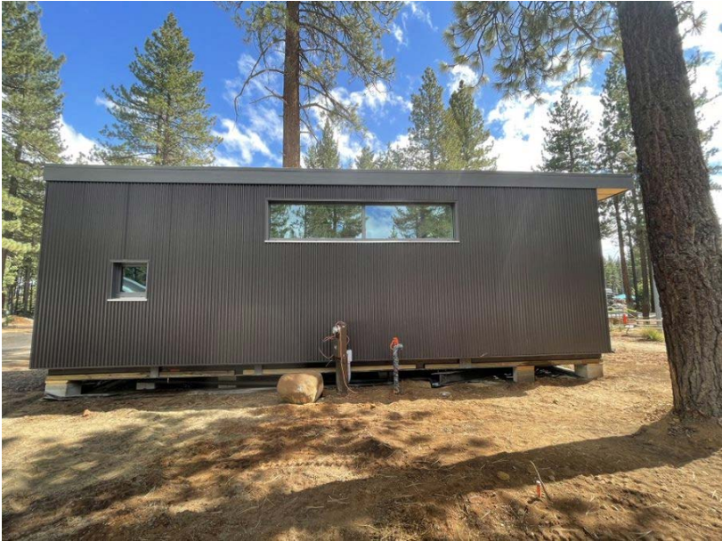
Figure 5. West side view of the test house
