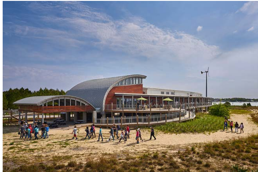
Chesapeake Bay Brock Environmental Center, Virginia Beach, Virginia. Photo from PNNL Distributed Wind Photo Gallery
