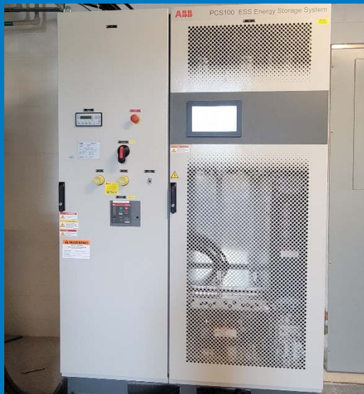
(a) Fuel cell inverter
