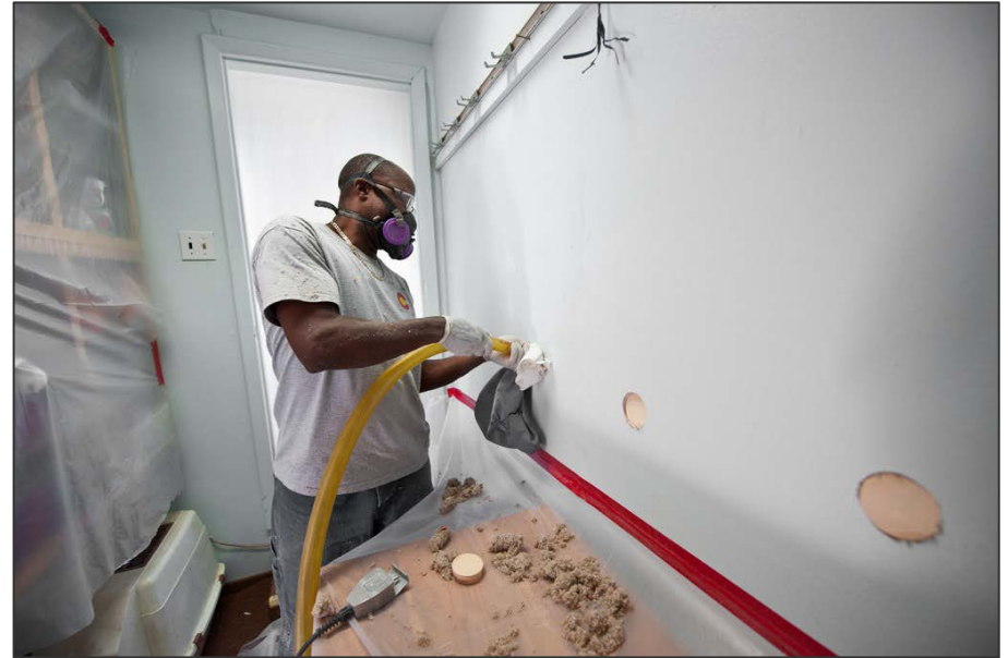
Photo from NREL image gallery 17963
