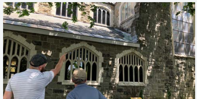
Retrofitting a historic library to be more energy efficient with help from C2C Expert Match. Photo from City of Cohoes
