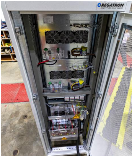
Fig. 5 Configuration of four Regatron GSS units as seen from the rear panel. (Photo by Werner Slocum, NREL)
