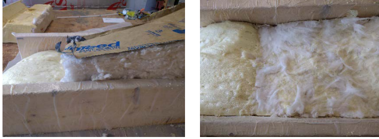
Figure 63. Injecting into fibrous insulation in open roof cavity
