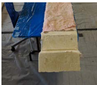
Figure 31. Foam fill at soffit
