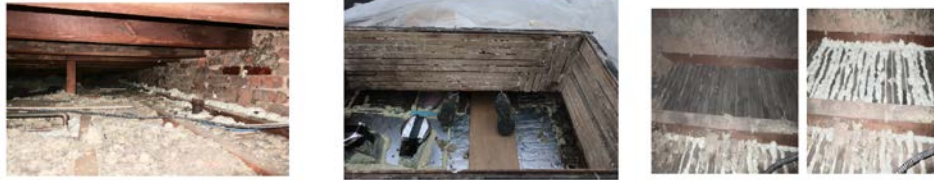
Figure 59. Air sealing triple-decker attics
