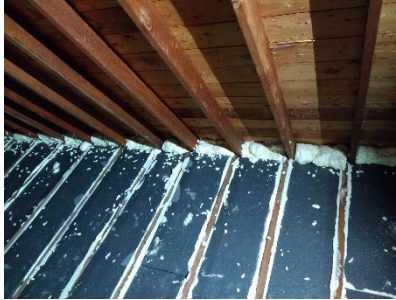
Figure 37. All cavities filled
