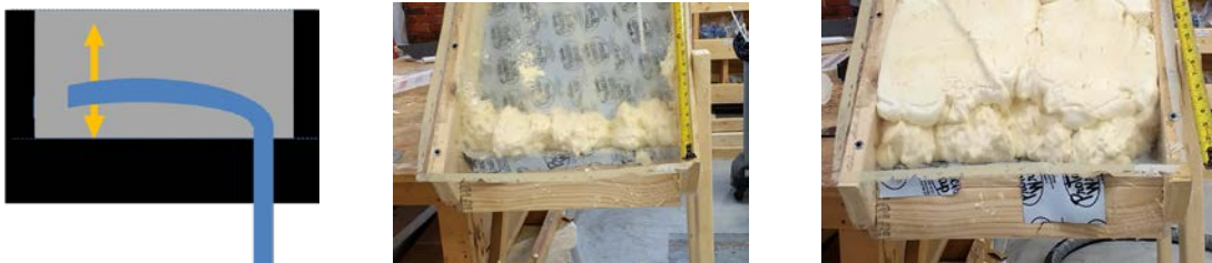
Figure 28. Top plate cross cavity dispense
