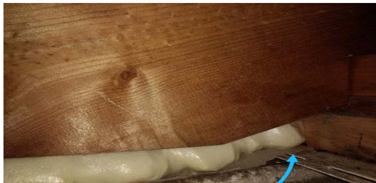
Figure 42. Paper liner in soffit
