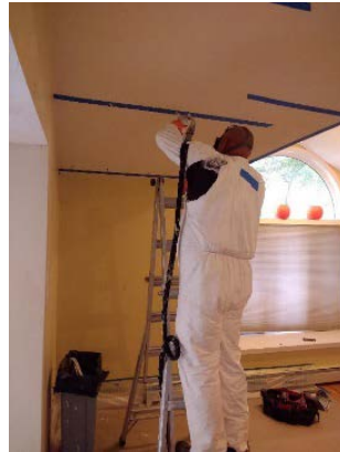
Figure 43. Injecting through the ceiling
