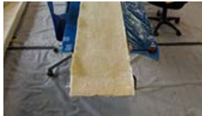
Figure 30. Foam fill at ridge vent
