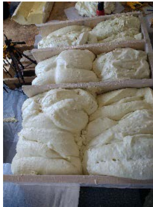
Figure 62. Open roof cavity with multiple rafter spacings
