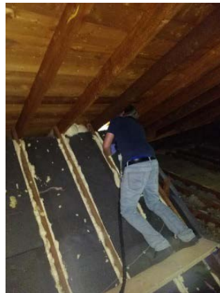
Figure 36. Injecting uninsulated cavity from the top
