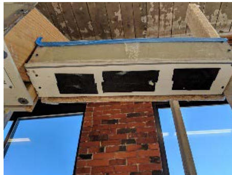
Figure 47. Pre-taped continuous soffit vent
