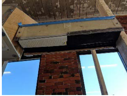
Figure 48. Pre-taped vinyl soffit vent
