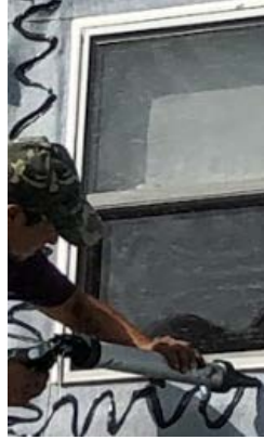
Figure 23. Liquid flashing sealing self-adhered flashing to rigid insulation
