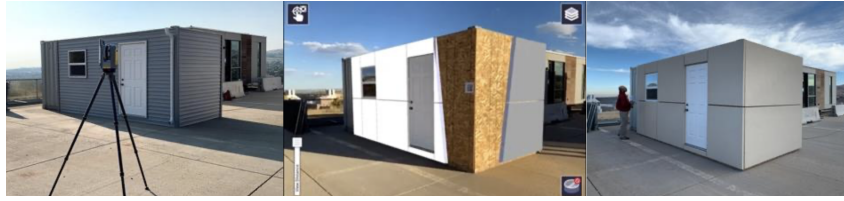
Figure 4: A two-sided test facade structure was constructed and scanned (left) for conversion into panel dimensions and manufacturing information, which were converted into a MR model for retrofit installation guidance (center) and ultimately the installation of the prefabricated over-clad retrofit (right).
