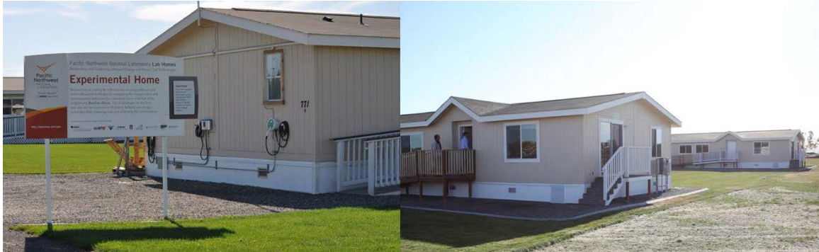
Figure 69. Exterior photos of the PNNL Lab Homes
