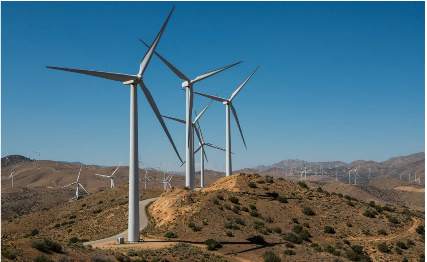
Pine Tree Wind and Solar Farm is part of NREL's 100% Renewable Energy Study. Photo by Dennis Schroeder, NREL 50710
