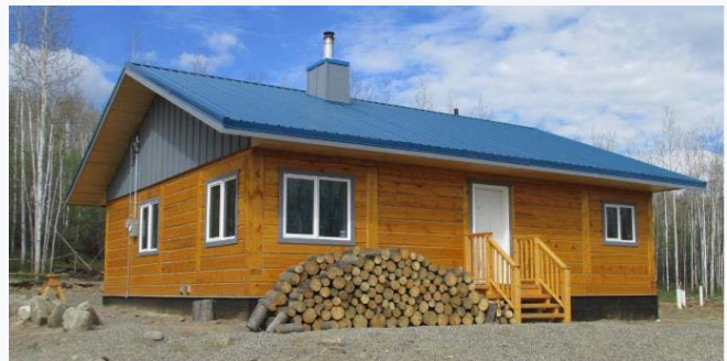
Prototype of the milled log kit home being developed by The Kuskokwim Corporation with NREL guidance. Photo from Dave Loeks, HTH Homes
