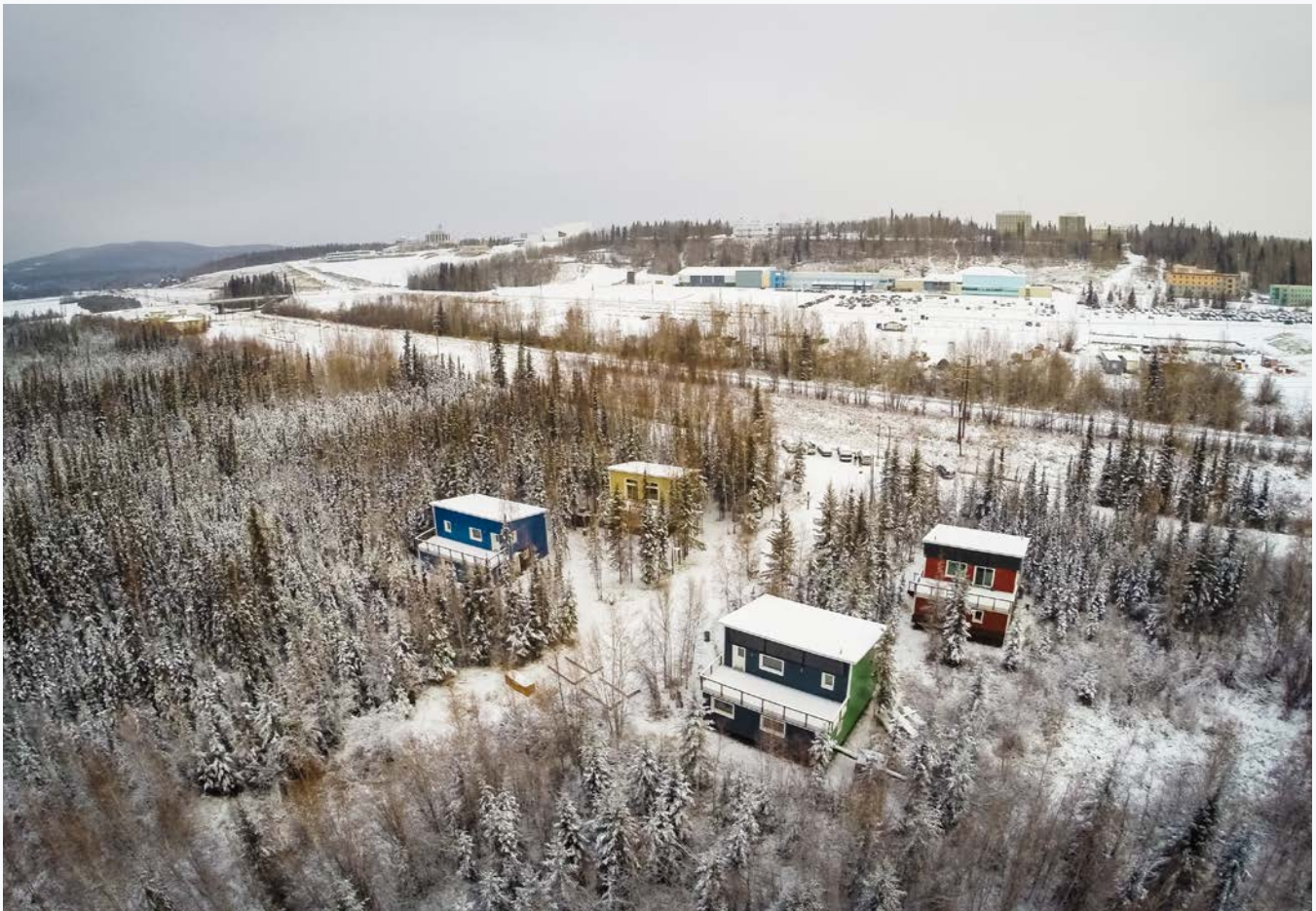
The Sustainable Village demonstrates a variety of building envelope, foundation, and heating approaches just outside NREL's Alaska Campus in Fairbanks. Photo by Seth Adams, NREL
