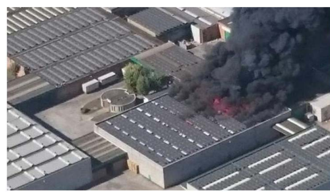
Example of PV fires in Italy. Fiorentini et. al., PVRW 2020. https://www.nrel.gov/docs/fy21osti/80055.pdf
