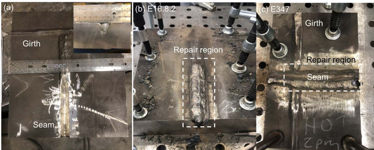
Figure 84. (a) Ground out single-V geometry form seam weld (b) after repair welding on seam weld using E16.8.2, and (c) after repair welding on seam weld using E347
