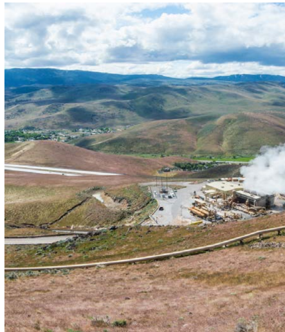
Photo Credit: Dennis Schroeder, NREL Steamboat Hills, Washoe County, NV
