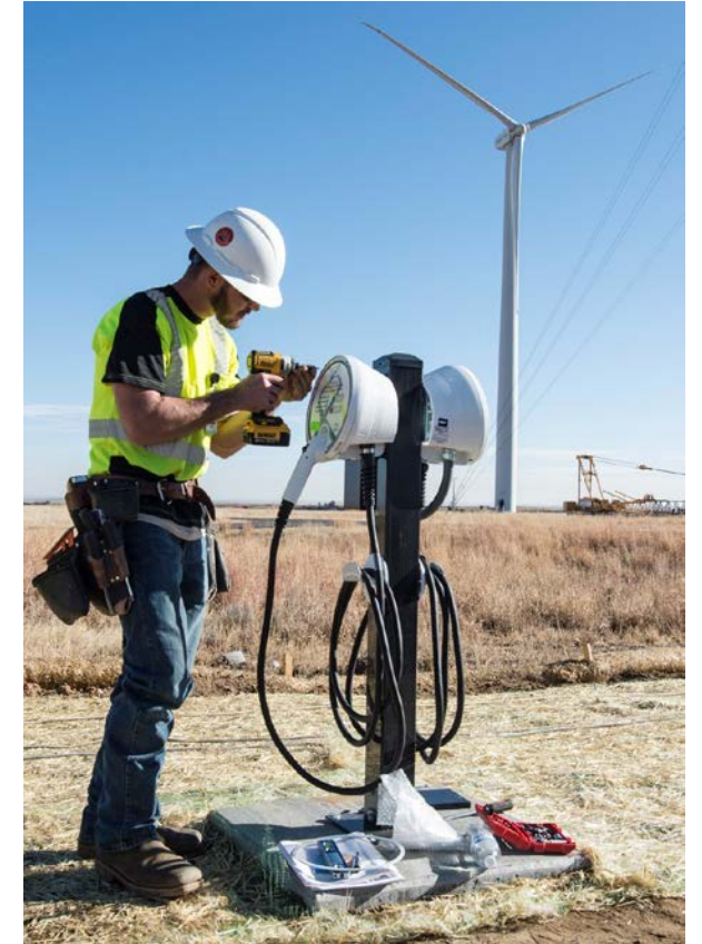
Installation of smart charging system at NREL's Flatirons Campus (Dennis Schroeder / NREL)
