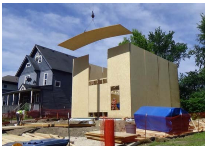
Figure 2. SPS home under construction
