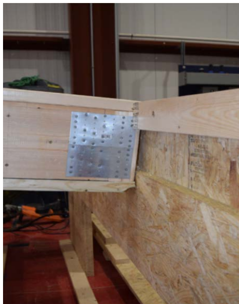
Figure A-14. Test 2 truss connection failure
