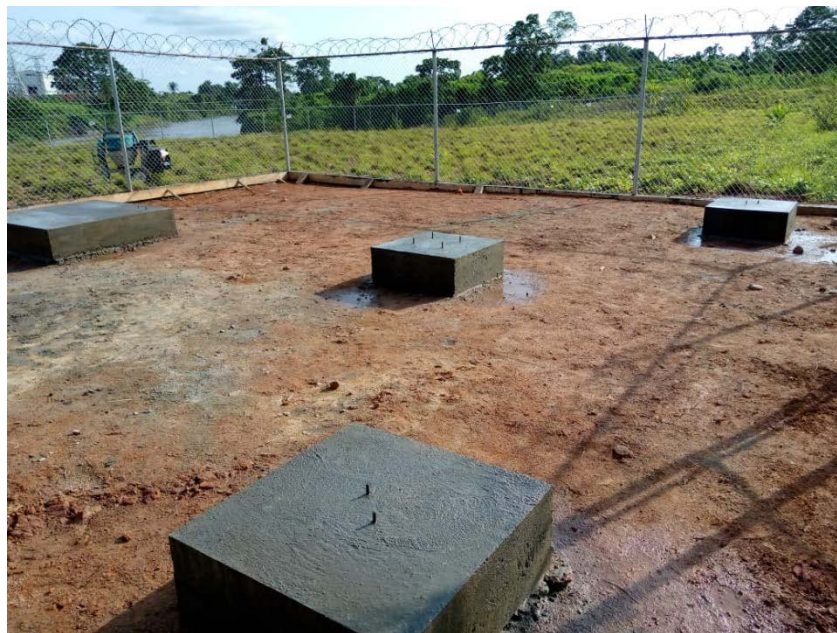
Figure 3A-9. Built foundations with threaded bolts.
