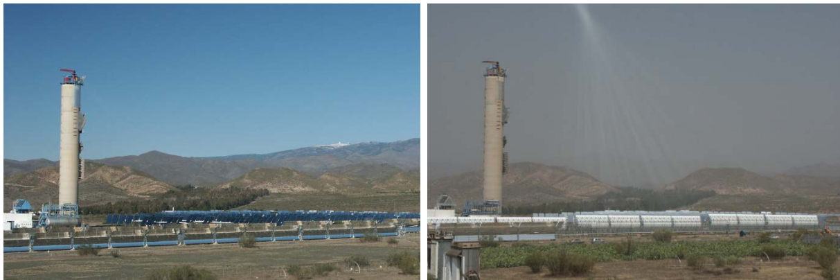
Figure 5-8. (Left) CIEMAT's CESA 1 solar tower on a clear day and (right) on a hazy day
