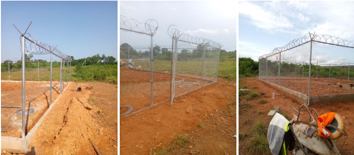
Figure 3A-8. Fence picture examples.
