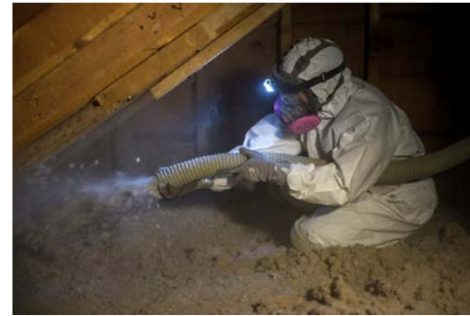
Installing attic insulation.
