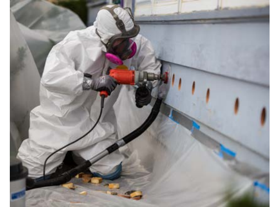
Installing exterior insulation.
