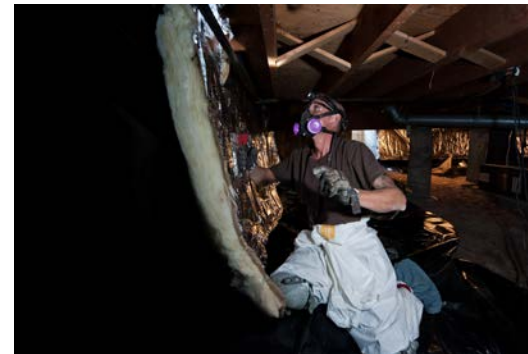
Installing crawlspace insulation.
