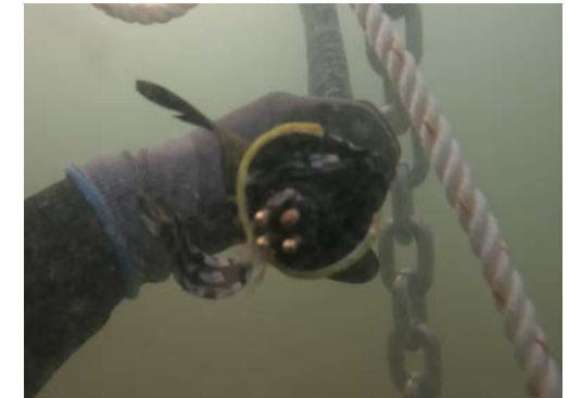
Load cell disconnected underwater
