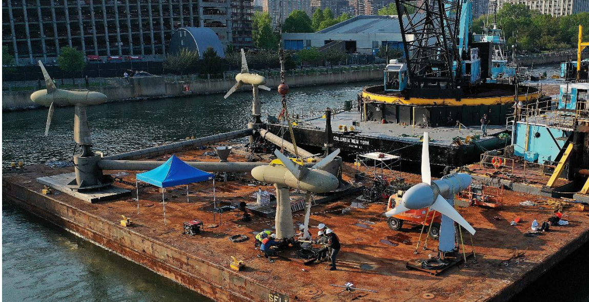
Figure 1. Photo showing the Verdant power retrieve-and-replace operation of their TriFrame at the RITE site with one fiberglass/epoxy rotor being replaced with the fiberglass/Elium rotor manufactured by NREL (photo by Paul Komosinski).
