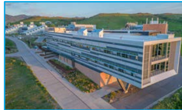
Energy Systems Integration Facility
