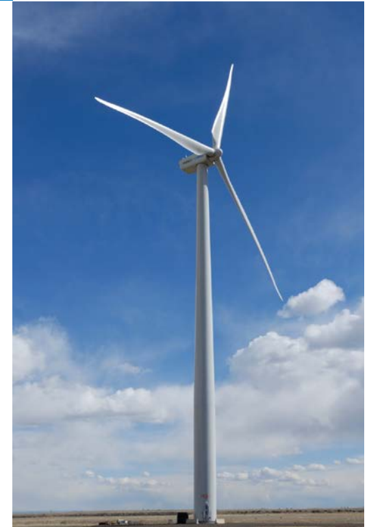
GE1.5 wind turbine located at NREL's Flatirons Campus. Photo by Jeroen van Dam, NREL
