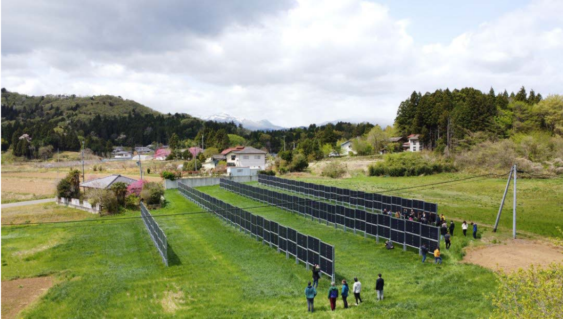
Figure 6. Vertical bifacial concept in Japan.
