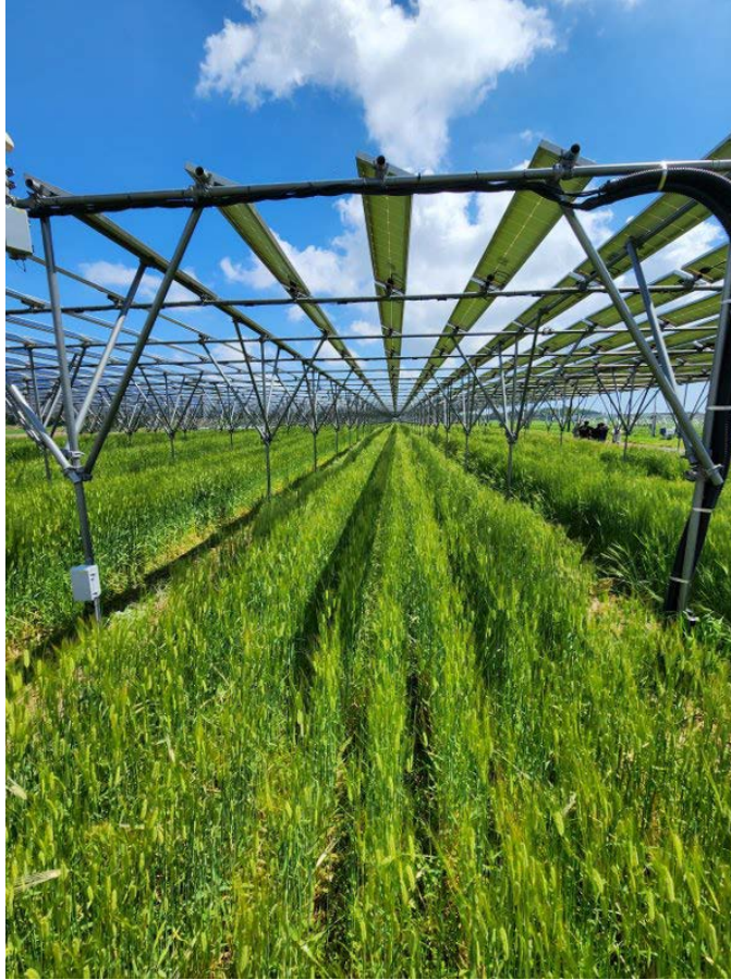
Figure 7. “Solar Sharing” concept in Japan.
