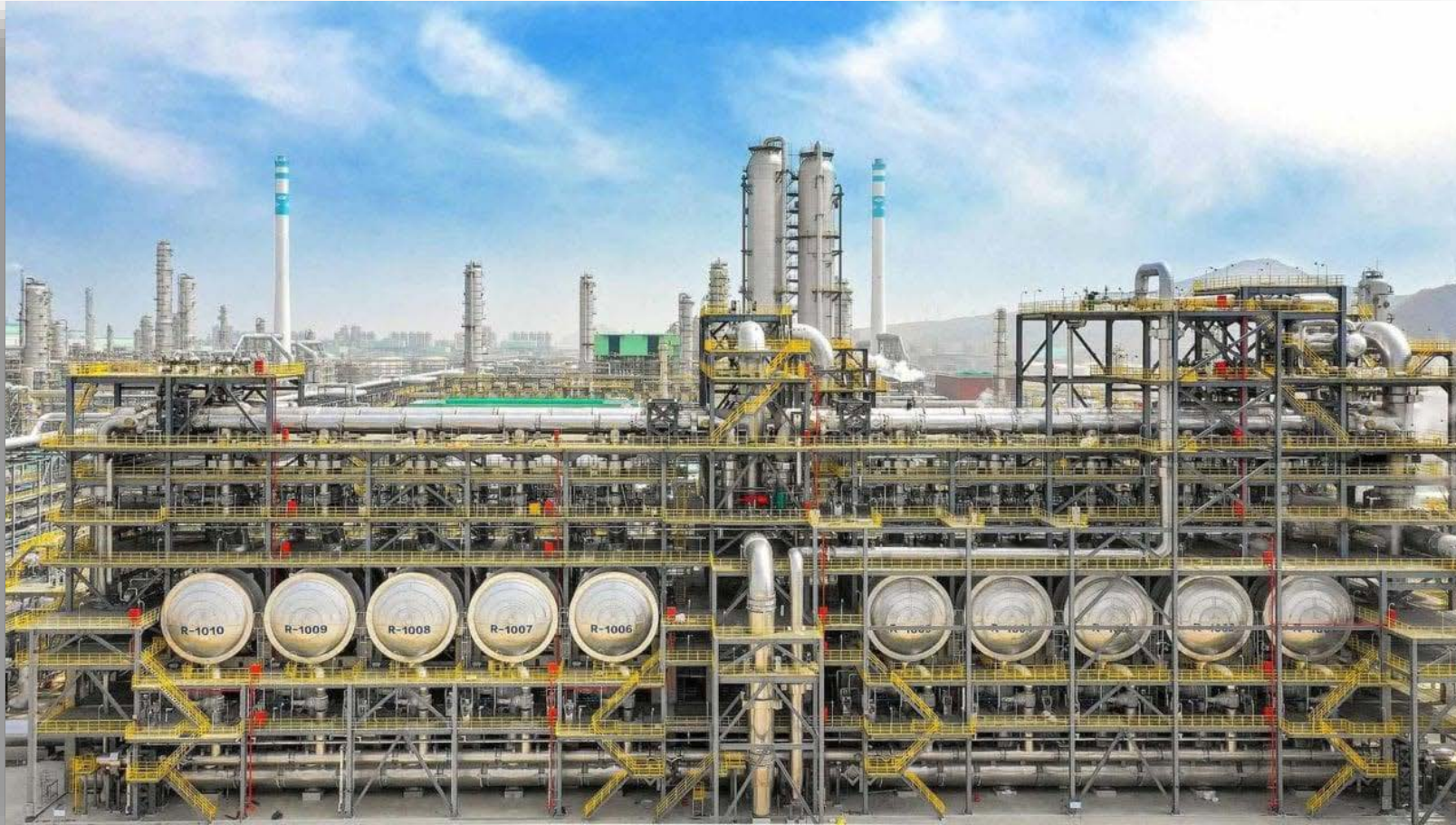
The world's largest Catofin plant for alkane dehydrogenation, Dalian, China (2019).
