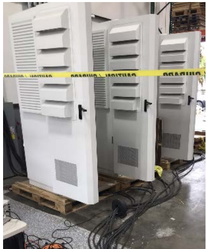
3000A of power converters-> to dispenser w/CAN dispatch control
