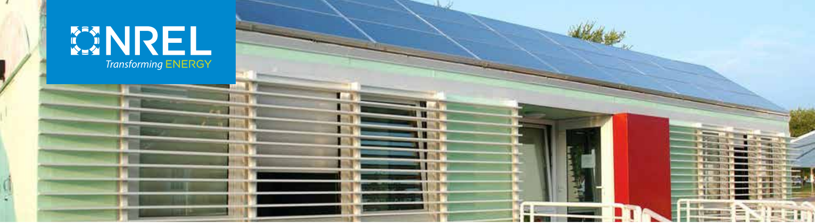
An energy-efficient house designed by the Puerto Rico team for the 2002 Solar Decathlon. Photo by Chris Gunn, NREL 12192
