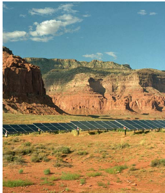
Photo by Warren Gretz, NREL
