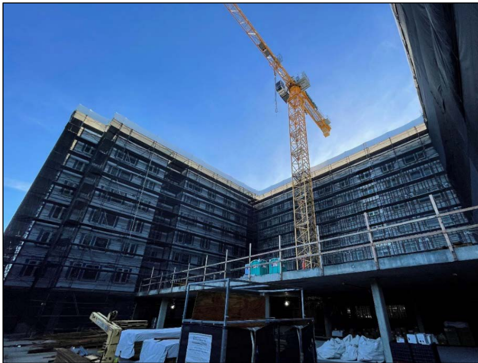
Figure 2. Site-built case study project in Seattle, Washington
