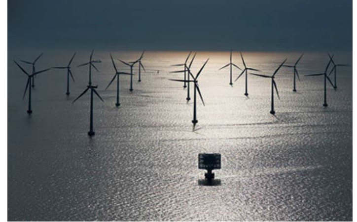
Lillgrund Offshore Wind Farm turbines and substation in Sweden.
