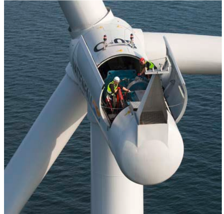
Maintenance is performed on a turbine at the Lillgrund Offshore Wind Farm in Sweden. Photo from Siemens AG, 27853
