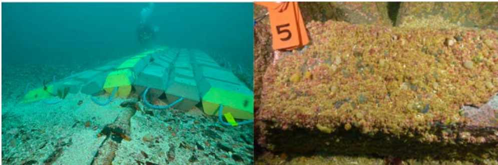
Newly installed concrete mattress over a partially exposed cable (left) and concrete mattress after it has been colonized by organisms after installation (right). Images from Taormina et. al (2020)
