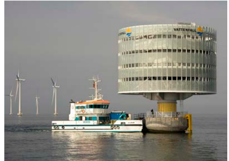
Maintenance is performed on a substation that is part of the Lillgrund Offshore Wind Farm in Sweden. Photo from Siemens AG NREL 27854.
