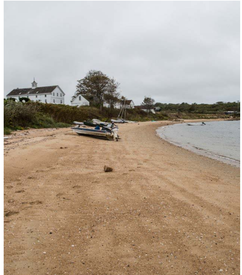
Block Island Wind Farm cable landing site. Photo by Dennis Schroeder, NREL 40394
